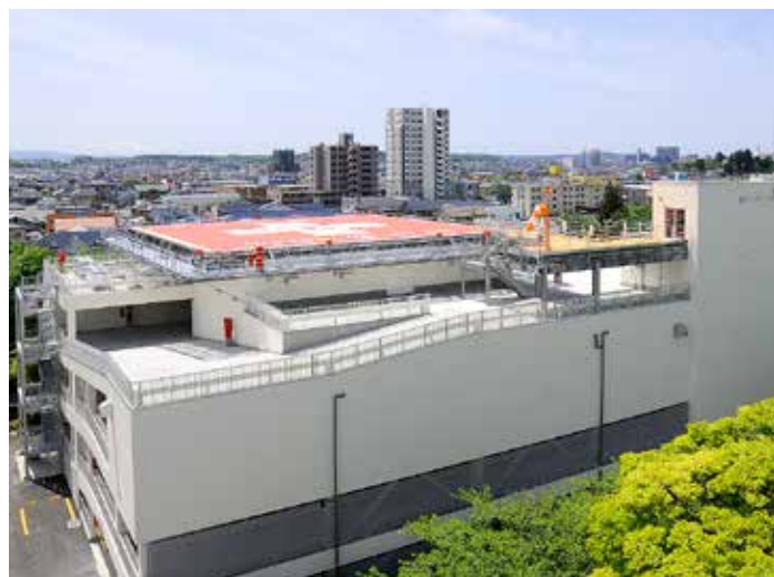
Helipad and Multistory parking lot
